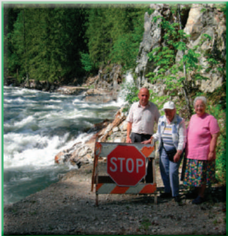
WASHED OUT SECTION OF ROAD AT CAR WASH FALLS SUMMER 2007
